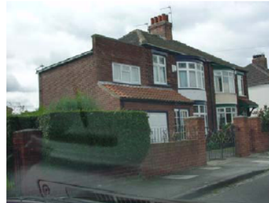
Fig D: Alien roof shape of extension destroys the balance of the house
